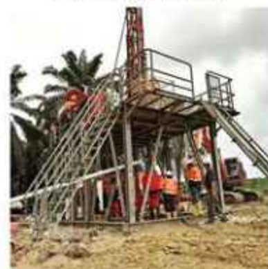
INDON CBM PTY LTD. CBM DRILLING
