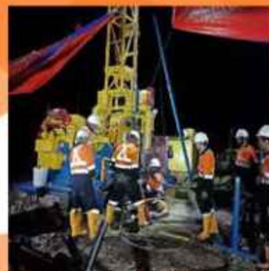
EPHINDO CBM DRILLING
