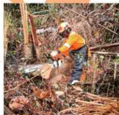
BHP BILLITON ACCESS PREPARATION
