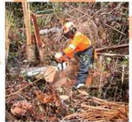
BHP BILLITON ACCESS PREPARATION
