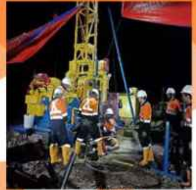
EPHINDO CBM DRILLING
