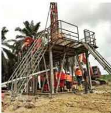
INDON CBM PTY LTD. CBM DRILLING
