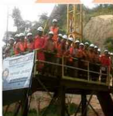
LEMIGAS CBM DRILLING
