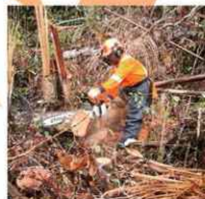
BHP BILLITON ACCESS PREPARATION
